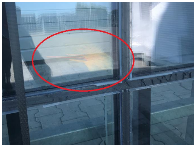
Fig. 32 Delamination of PVB film due to chemical incompatibility
