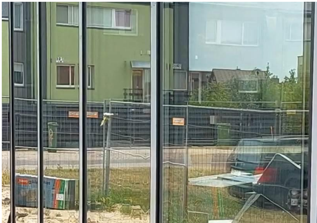
3 Fig. Based on influence of the overall bow and roller waves, a slight "waving" effect is permissible, which has no view disturbing when observing perpendicularly the main area of the glass
