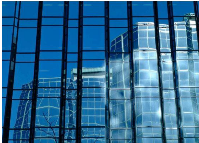
Fig. 26 Distortion effect, depending on concavity/convexity of glass panes due to overall bow and roller wave of toughened glasses, etc.
