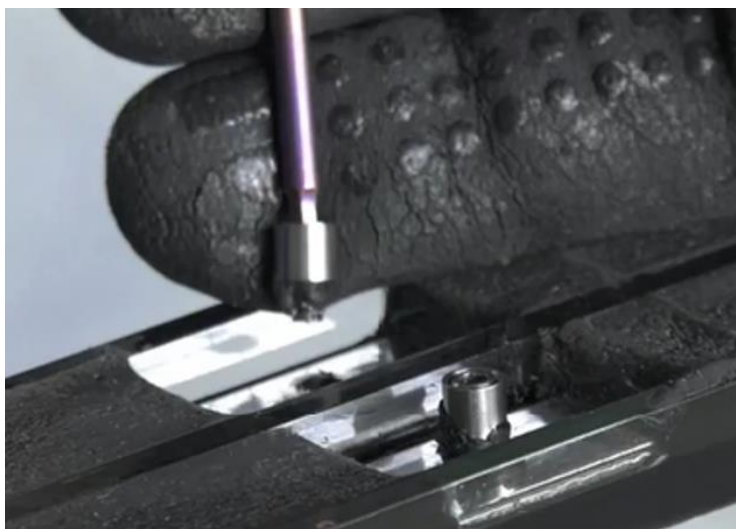
Fig. 13 SWS Air installation into insulating glass unit
