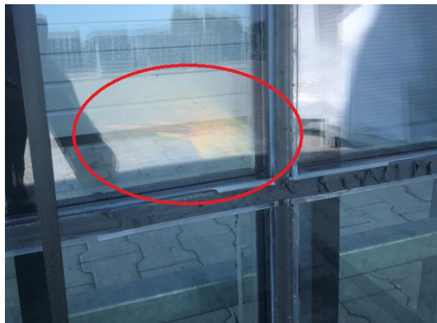
Fig. 35 Delamination of PVB film due to chemical incompatibility
